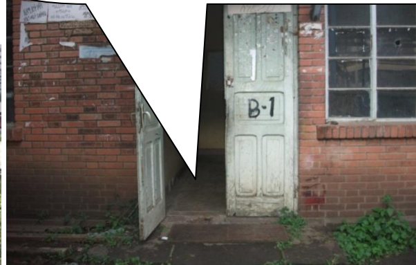
Figure 4.12: The existing high edge at the entrance of Mini Media causes inaccessible for students using wheelchair at Menelik II Primary School
