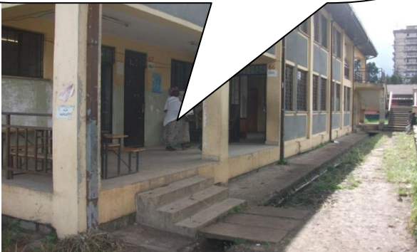
Figure 4.11: The stairs and high edges make administrative offices inaccessible for students using wheelchair at Menilik II Primary School
