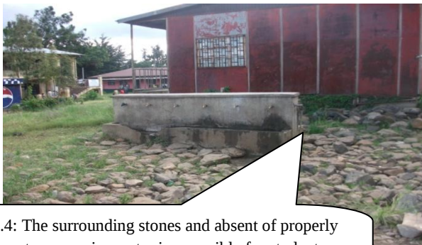
Figure 4.5: The existing edge and hole for drained water in the vicinity of the pipe water causes inaccessible for students using wheelchair at Menelik II Preparatory School
