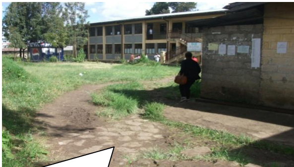
Figure 4.2: The physical condition of Menelik II Primary School.
