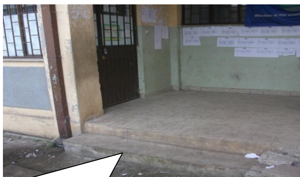
Figure 4.9: The stairs causes inaccessibility Science Laboratory for students using wheelchair at Menelik II Primary School
