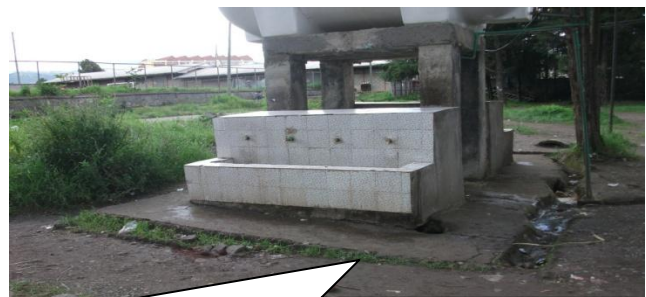
Figure 4.5: The existing edge and hole for drained water in the vicinity of the pipe water causes inaccessible for students using wheelchair at Menelik II Preparatory School
