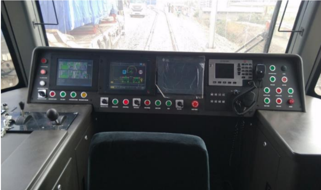
FIGURE 17: THE INTERIOR OF THE CAB
