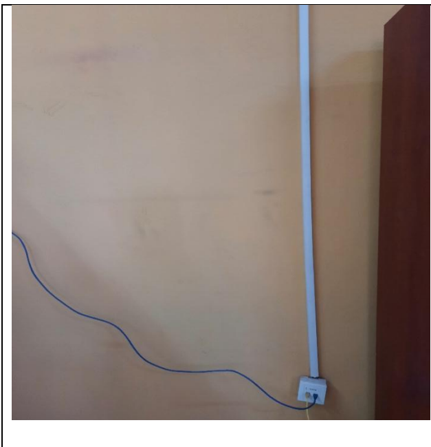
Figure 4.7: Photo showing external data and electrical lines
