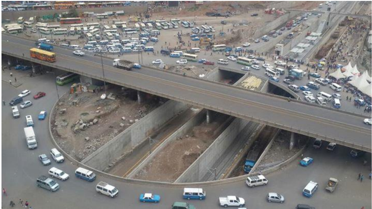
Figure 4.8.3.2: New road construction in Addis Ababa at Megenagna
