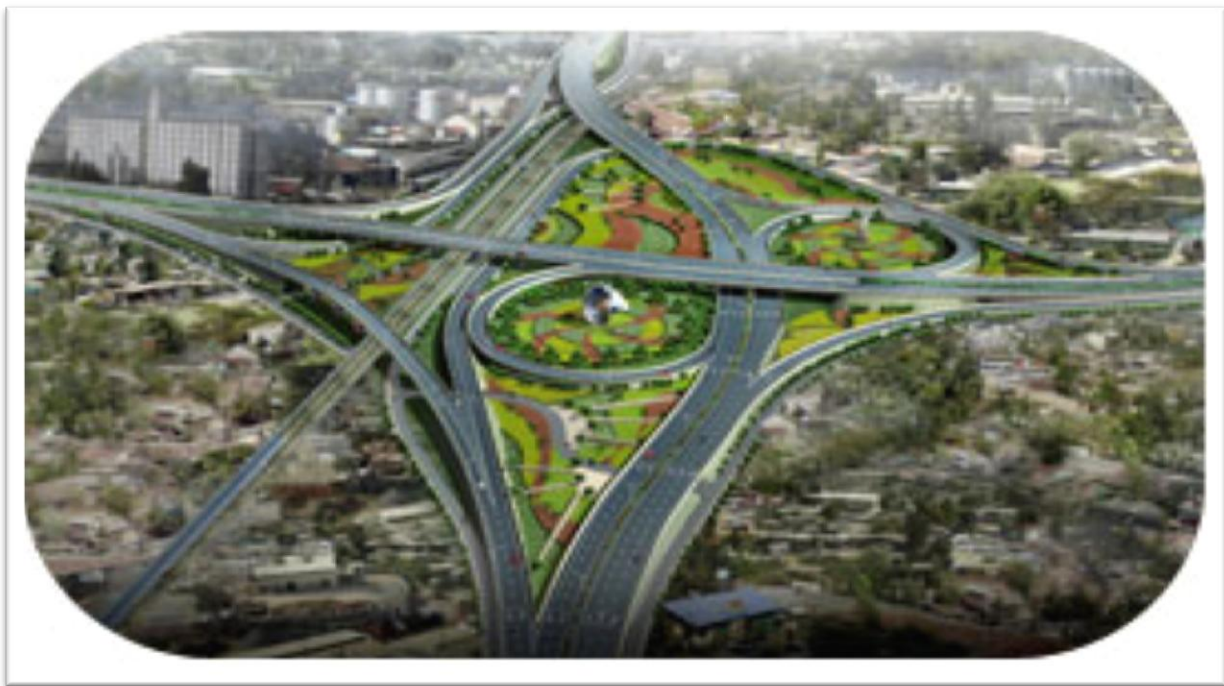
Figure 4.8.3.1: Road construction in Addis Ababa Gotera Interchange
