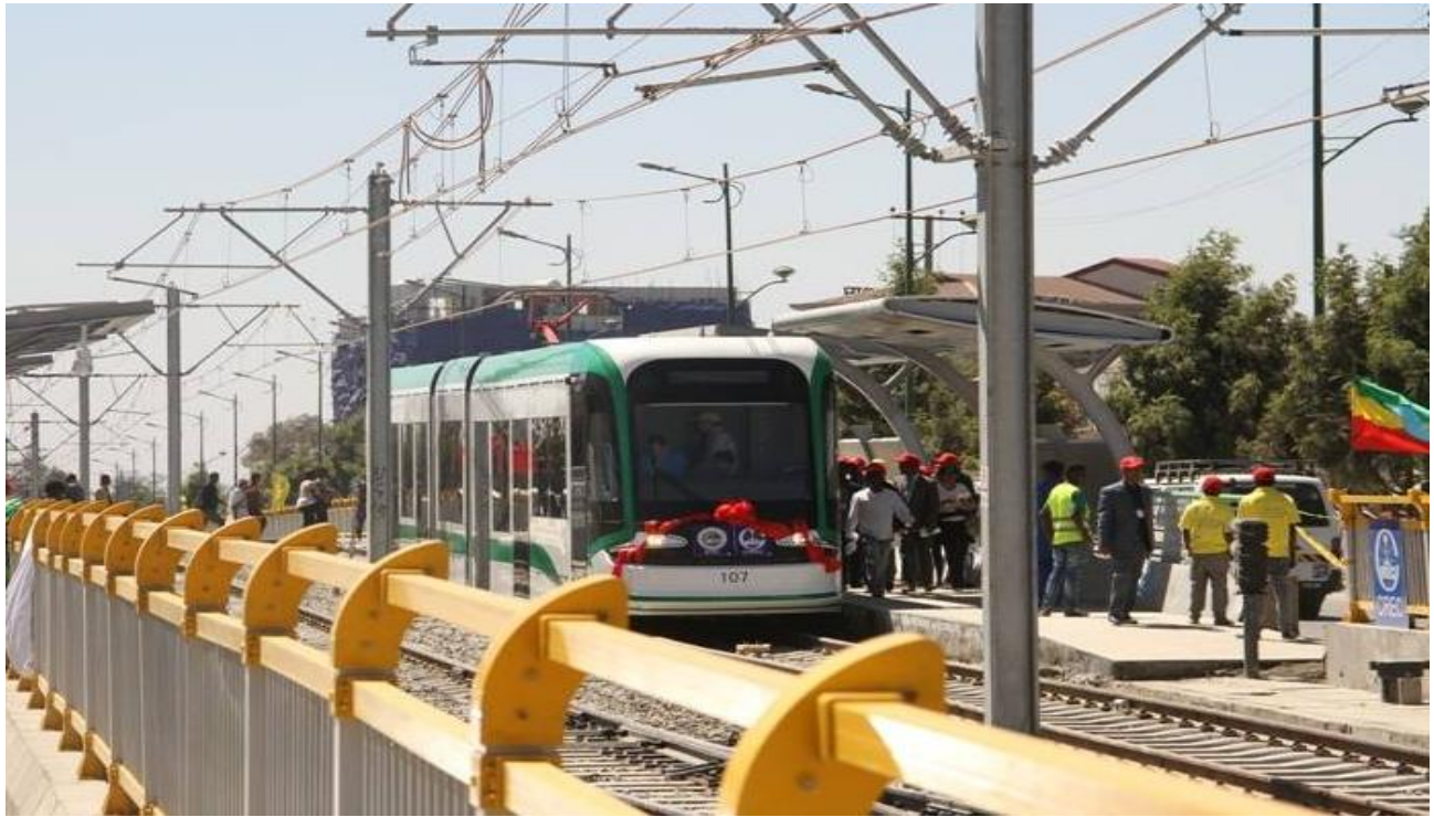
Figure 6.1B: Ongoing railway construction in Addis Ababa
