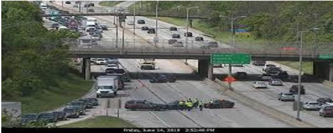
Figure 2.4 Over pass bridge. Source: Google
