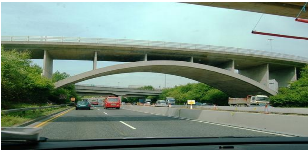
Figure 2.5 over Pass Bridge. Source: Google
