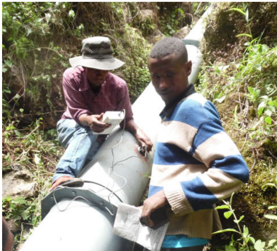
Fig.3. 6: Flow Velocity Reading on the site during the test
