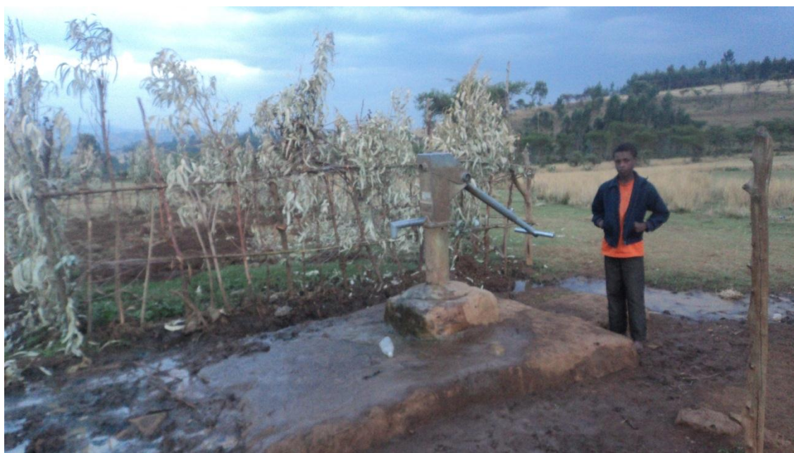
Figure 6-2 Photo taken during field work sanitation problem scheme
