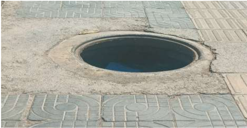
Image for Figure 1: uncovered pipes in road around work place
