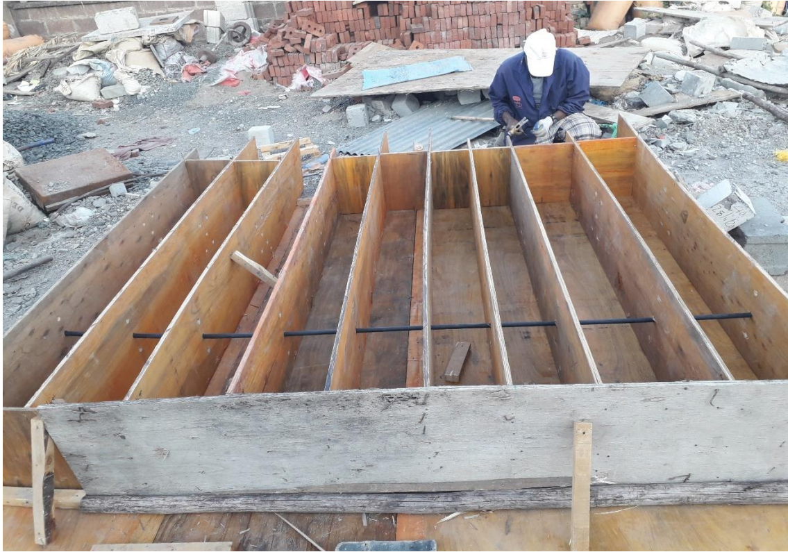
Figure 3-11: Formwork Assembly for Main Specimens
