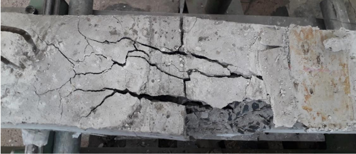
Figure 4-22: Top Longitudinal Cracking (SII10-50)
