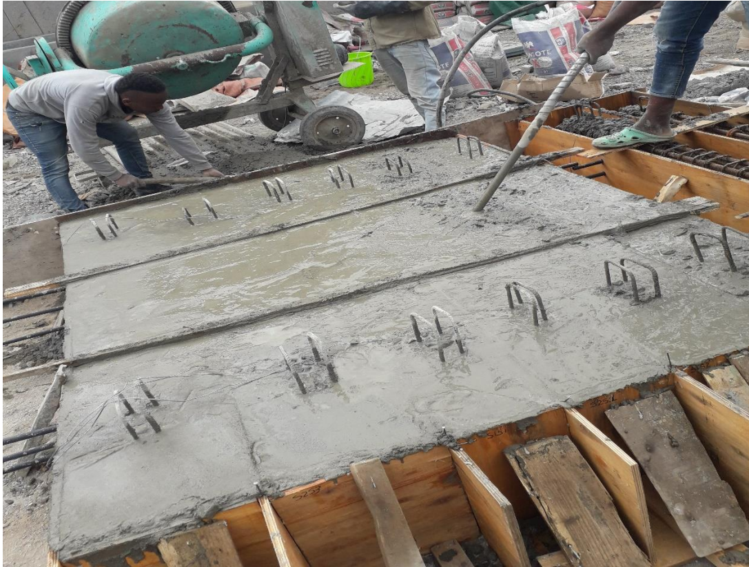
Figure 3-19: Concrete Casting of Main Specimens
