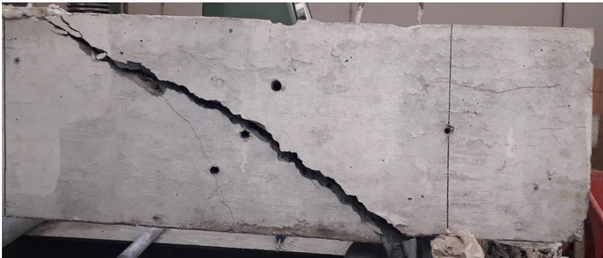
Figure 4-29: Diagonal Compression Crack at Failure Front Side (SIII10-75)
