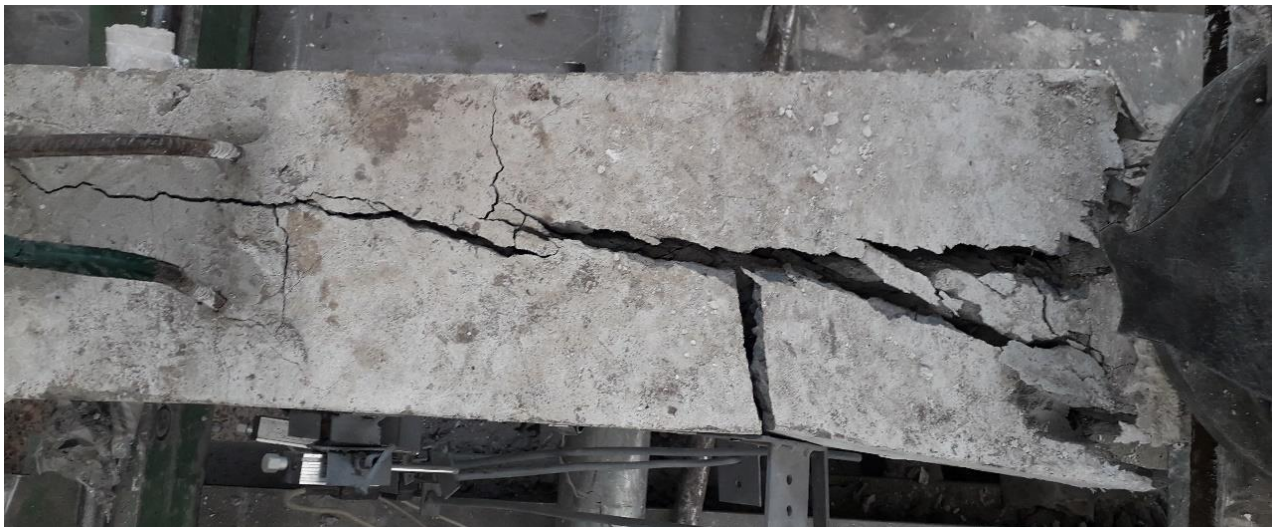
Figure 4-3: Top Longitudinal Crack at Failure (TRIAL Beam (TR 8-50/75))
