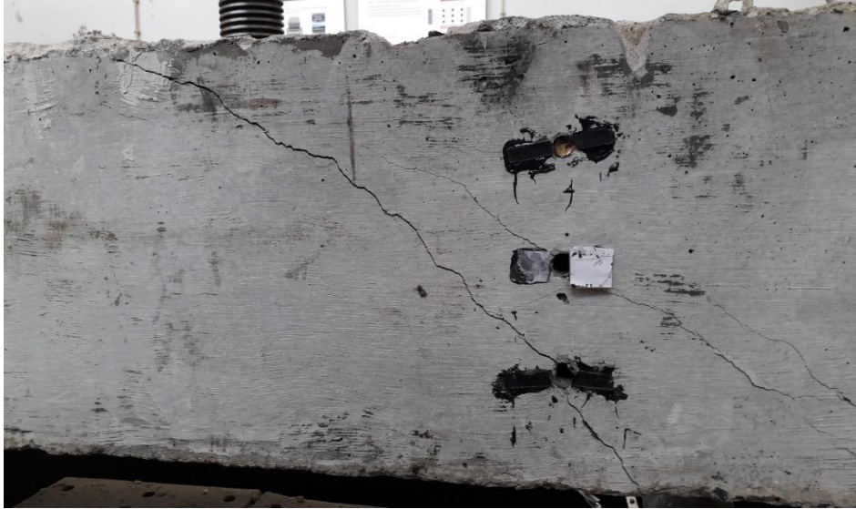
Figure 4-44: Diagonal Compression Crack at Failure Back Side (SIII0-75)
