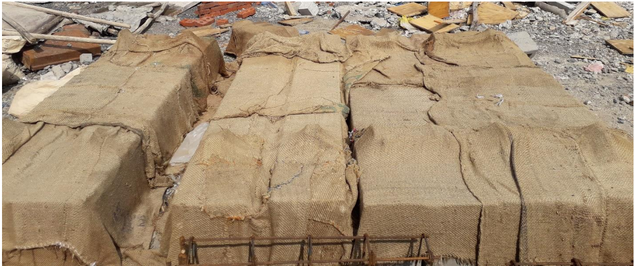
Figure 3-21: Main Specimen Curing
