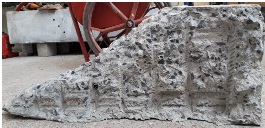
Figure 4-34: Spalled Piece of Side Cover (SIII10-75)
