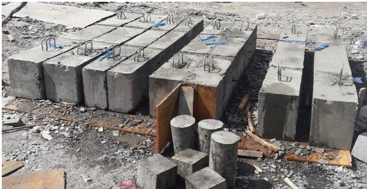
Figure 3-20: Formwork Removal of Main Specimens
