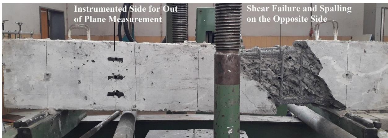
Figure 6-15: SII10-50's Failure Opposite to the Instrumented Side
