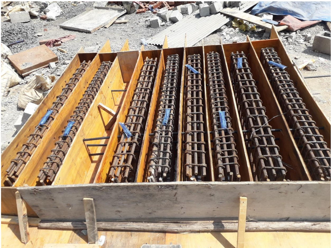
Figure 3-17: Reinforcement Cage Placed in Formwork (Main Specimens)
