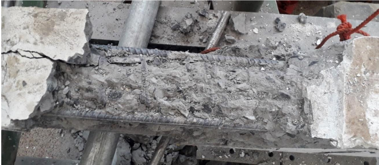
Figure 4-8: Side Cover Spalled, Top View (TRIAL Beam (TR 8-50/75))
