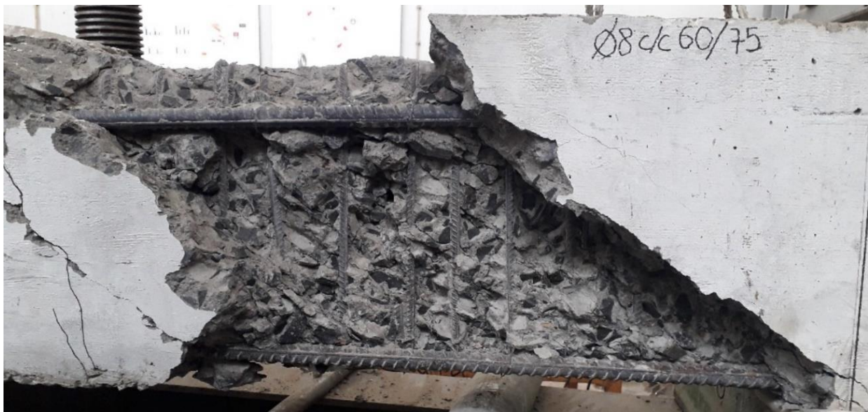
Figure 4-7: Side Cover Spalled, 75 mm Side Cover (TRIAL Beam (TR 8-75))
