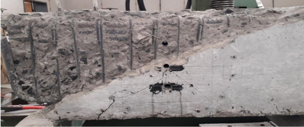
Figure 6-29: Spalling on One Side of the Beam Above the Diagonal Crack
