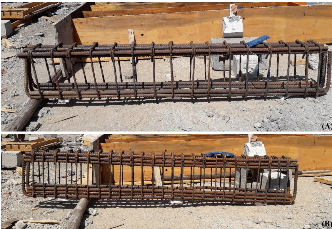
Figure 3-13: Reinforcement Cage for Main Specimens (A) SIII0-25 (B) SIII8-75
