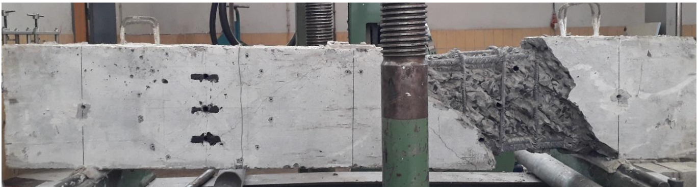
Figure 4-27: Final State of Beam After Failure (SIII10-50)
