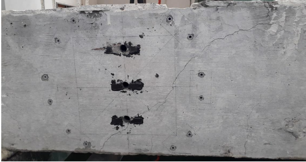
Figure 4-46: Diagonal Compression Crack at Failure Front Side (SIII0-75)
