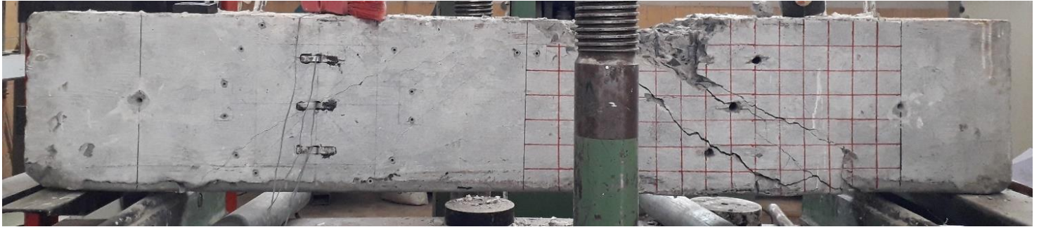
Figure 4-20: Final State of Beam After Failure (SI8-50)
