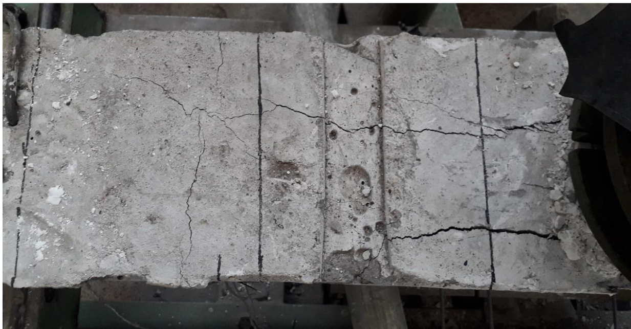
Figure 4-11: Top Longitudinal Crack (SI8-25)
