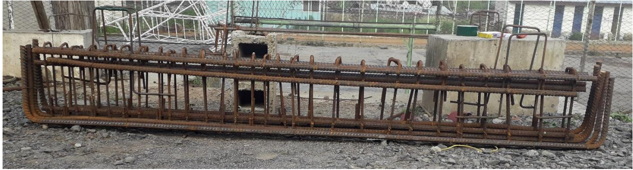
Figure 3-12: Reinforcement Cage for Trial Beam
