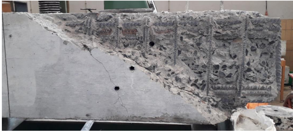
Figure 4-33: Spalled Section Front Side (SIII10-75)
