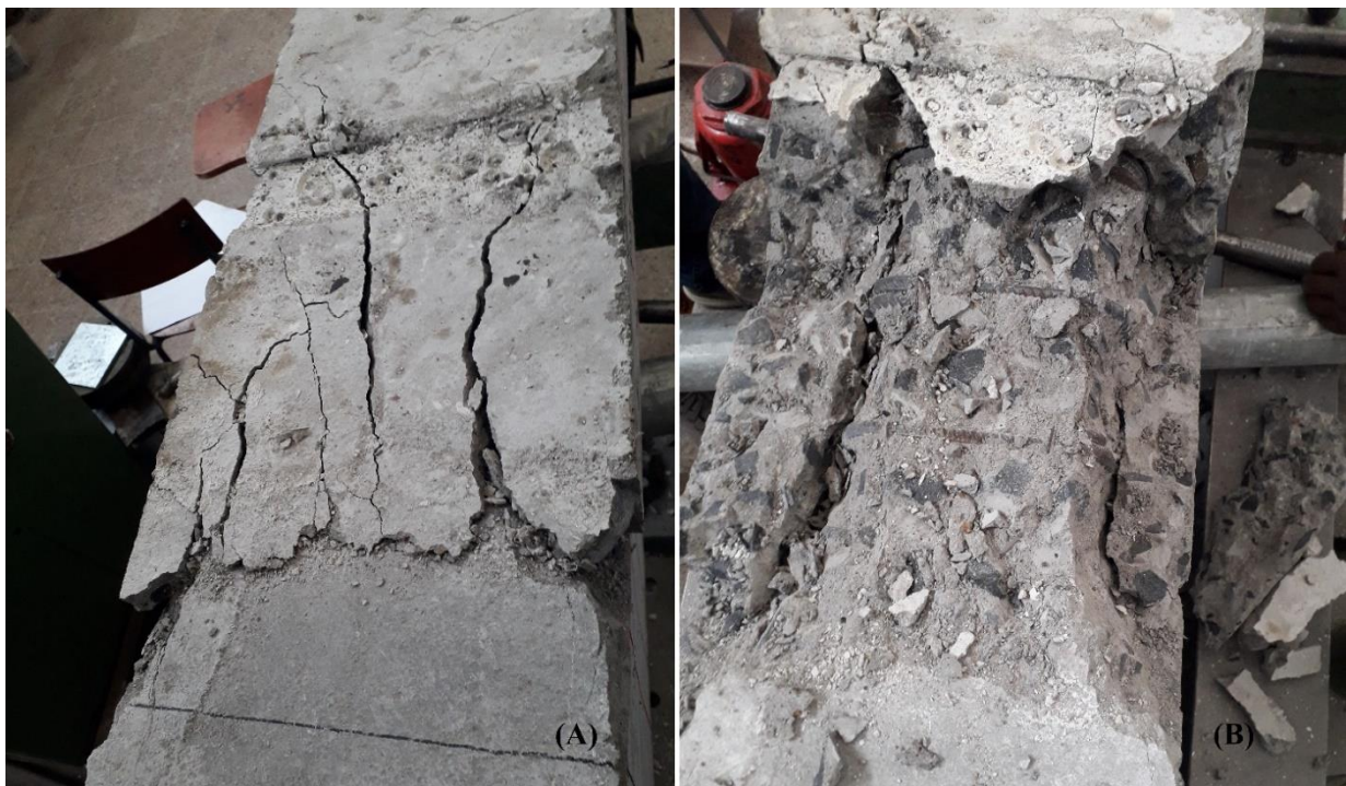
Figure 4-17: (A) Top Longitudinal Cracking (B) Spalled Section Top View (SI8-50)
