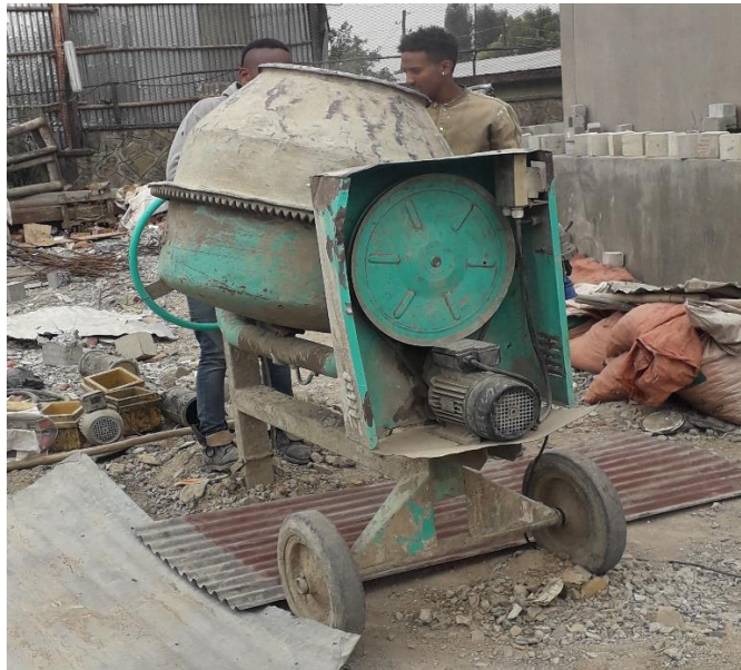
Figure 3-18: Tilting Drum Mixer used for Concrete Casting
