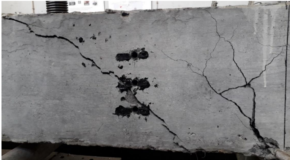
Figure 4-40: Diagonal Compression Cracks at Failure Back Side (SIII8-75)
