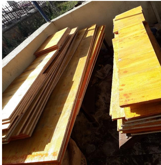
Figure 3-10: Plywood used for Formwork Construction
