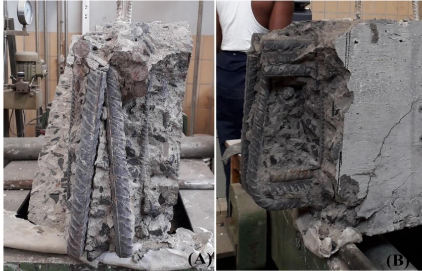
Figure 4-32: (A) Spalling on the Rear End of the Beam (B) Spalled Section Back Side (SIII10-75)
