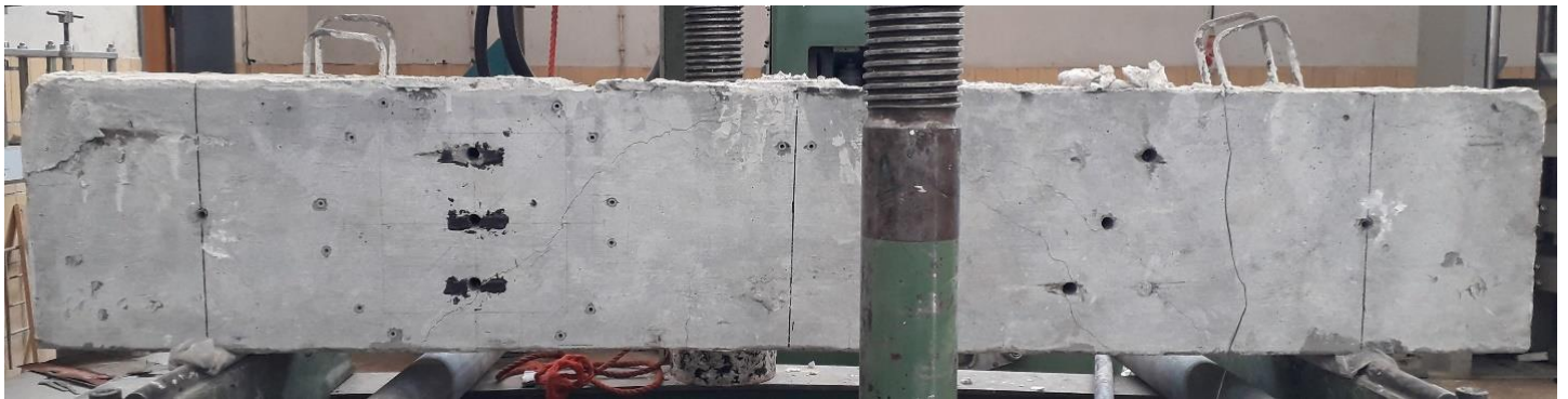
Figure 4-47: Final State of Beam After Failure (SIII0-75)
