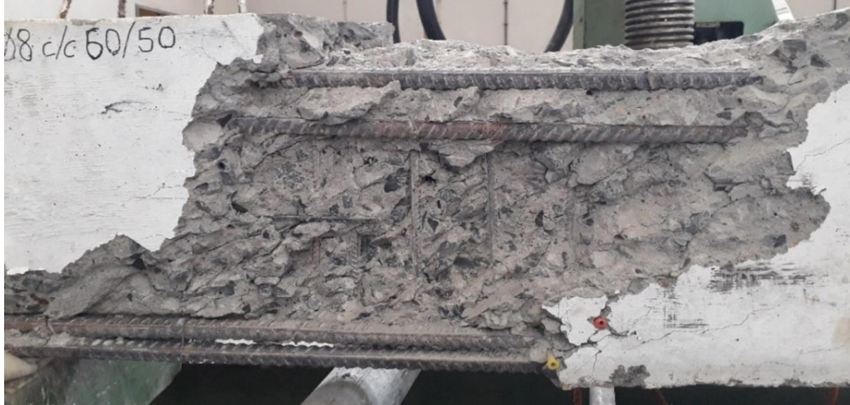
Figure 4-6: Side Cover Spalled ,50mm Side Cover (TRIAL Beam (TR 8-50))
