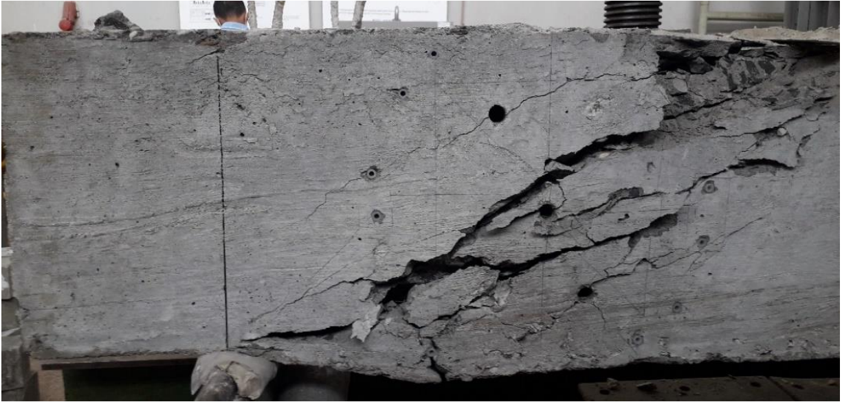
Figure 4-24: Diagonal Compression Crack and Top Spalling at Failure Back Side (SII10-50)
