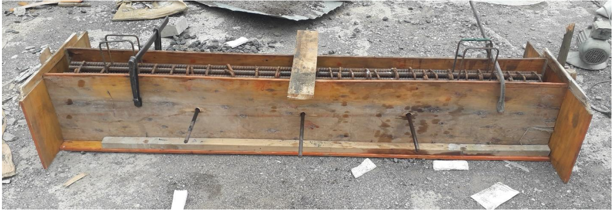
Figure 3-16: Reinforcement Cage Placed in Formwork (Trial Beam)
