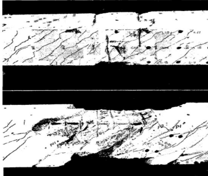
Figure 2-4: 1974, Mitchell and Collin Beams PT5 and PT6 at failure
