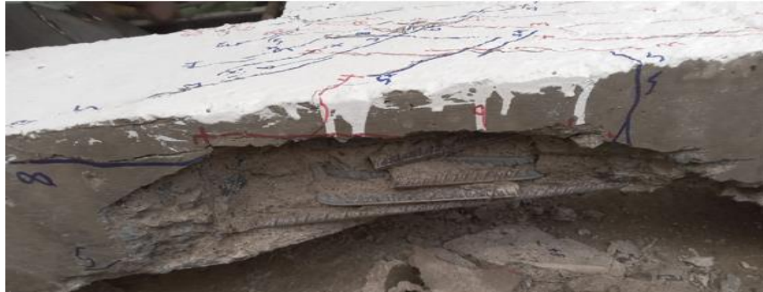
Figure 4:1: joint shear failure in Specimen Bcj-9.5-sv
