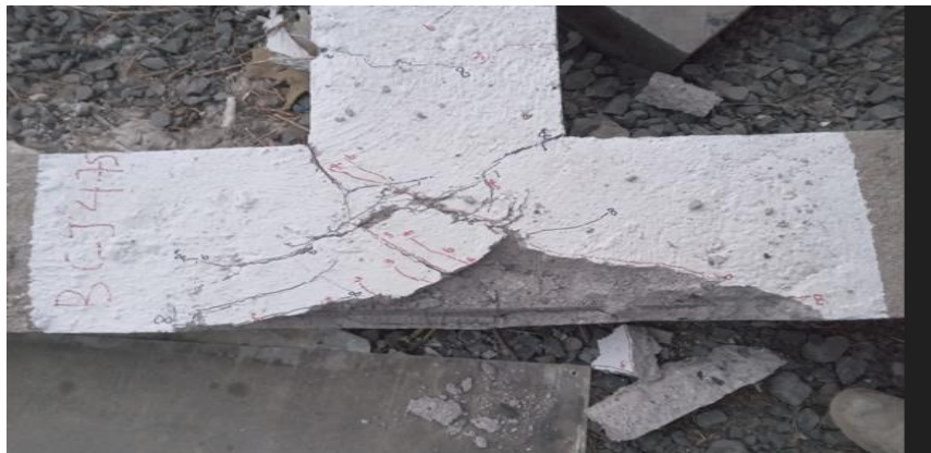
Figure 4.2 joint shear failure in Specimen Bcj-4.7
