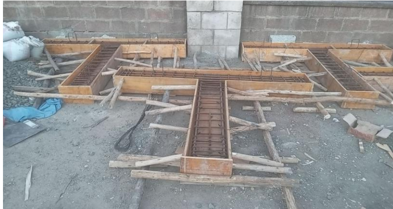
Figure 3.5: Reinforcement cage and formwork of the specimens
