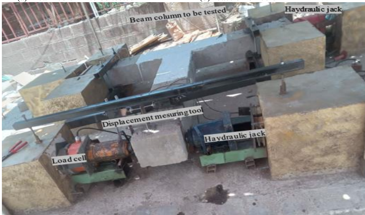
(c) Full prepared beam column joint for test
