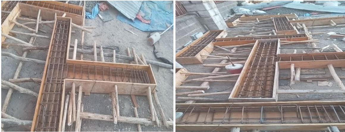
Figure 3.6: Reinforcement cage of specimens inside the formwork
