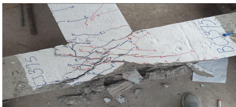
Figure 4.5 joint shear failure in Specimen Bcj-37.5
