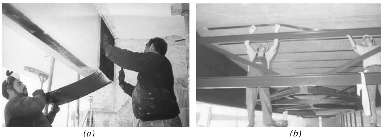
Figure 2-3: Basic FRP EBR Application Technique (FIB 14)
