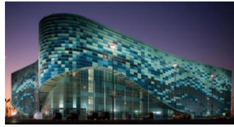
The Iceberg Skating Palace, Sochi, Russia Aluminium was one of the key materials used to the construction.
