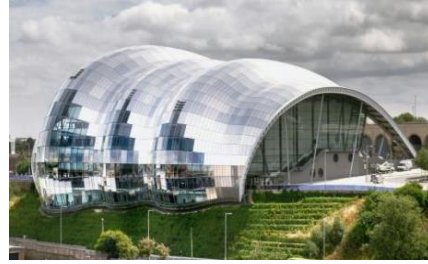
The Sage Gateshead, Gateshead Quays, UK Al was used to support the glazing system
