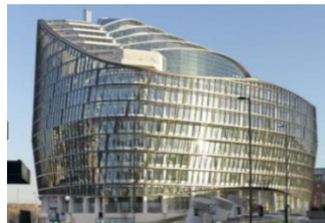
The Co-operative Group, Manchester, UK The anodised exterior aluminium structure holds the glass panels.
