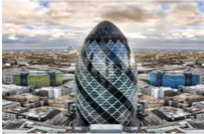
St Mary Axe, London, UK A curved and anodised aluminium skin was used to integrate the raking columns with the curve façade
