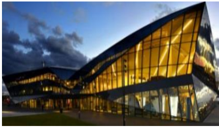
The Crystal, London, UK The roof is made from 100% recycled aluminium
