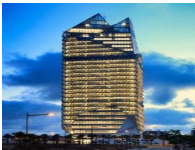
Casablanca Finance City Tower, Casablanca, Morocco The modular façade elements were made out from aluminium instead of concrete for cost reasons.
