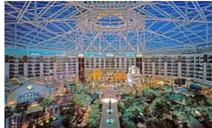
Gaylord Texan Resort & Convention Center, Grapevine, Texas, USA The roof is made of a glazed aluminium framework
