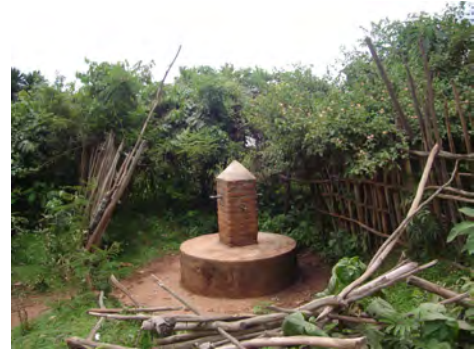
Figure 3-3: Typical underground (with two taps) and above ground (four taps) water Points
