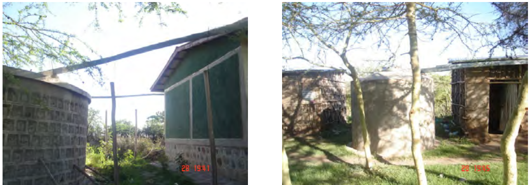
Figure 5-3: 150 m 3 Masonry and 10 m 3 Ferro Cement Reservoir In Kiticha primary Second cycle School
