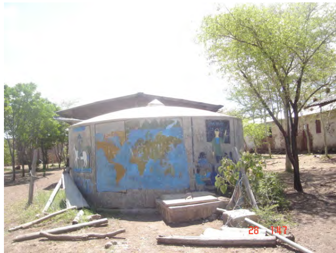
Figure 1-1: Typical 40 M 3 Ferro Cement Reservoirs in Chele Primary Second Cycle School, Minjar and Shenkora Woreda
