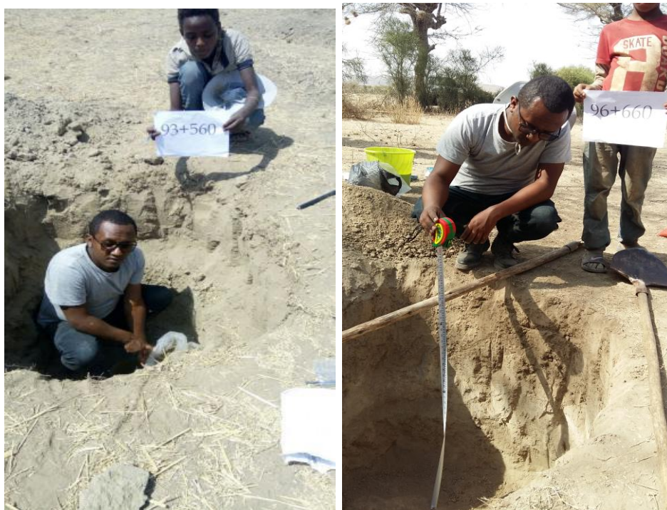
Figure 11: Test pits dug at km 93+560 and km 96+660
