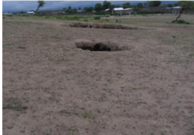
Figure 2: Collapse holes near Shashemene (Source: ERA Site Investigation Manual)
