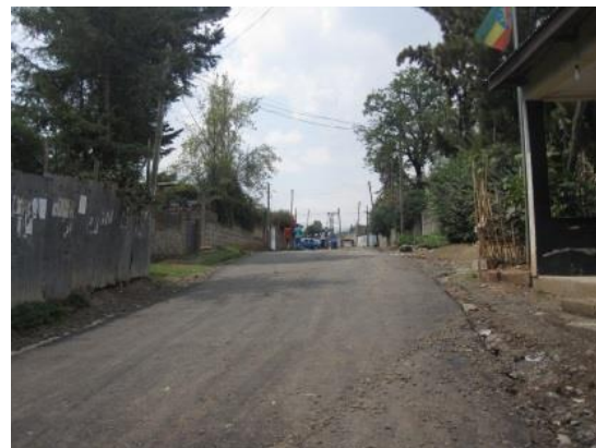
Figure 3.20: Paved road to Enderase
