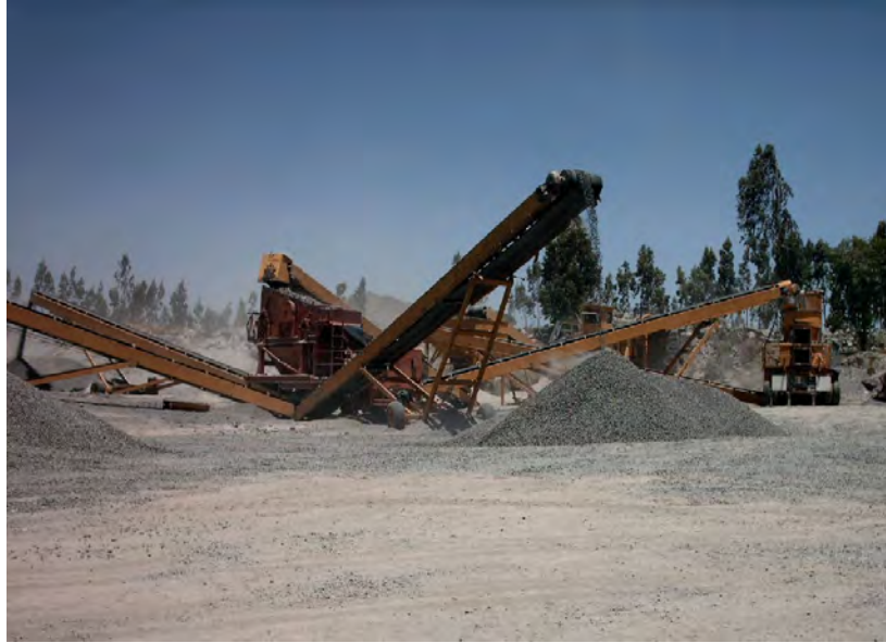
Fig 3.6 Large scaled coarse aggregate production plant (Blue Nile -around Kaliti)
