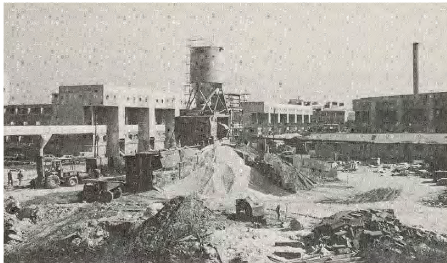
Fig 2.6 Aggregate for concrete stored in a mixing area [7].
