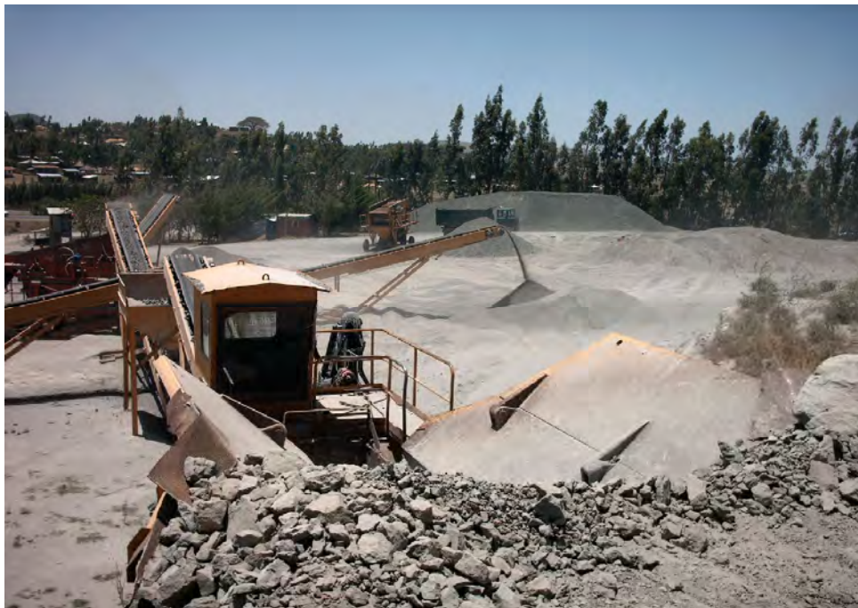
Fig 3.7 Dust produced by a process of coarse aggregate production (Blue Nile)
