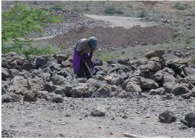
Fig 3.4 Boulders for coarse aggregate preparation being crushed by human labor.
