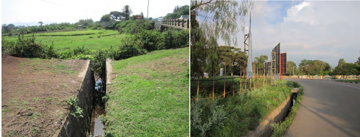
Figure 20 Main drainage lines which end up in to Lake Hawassa (Source: field survey March, 2013)
