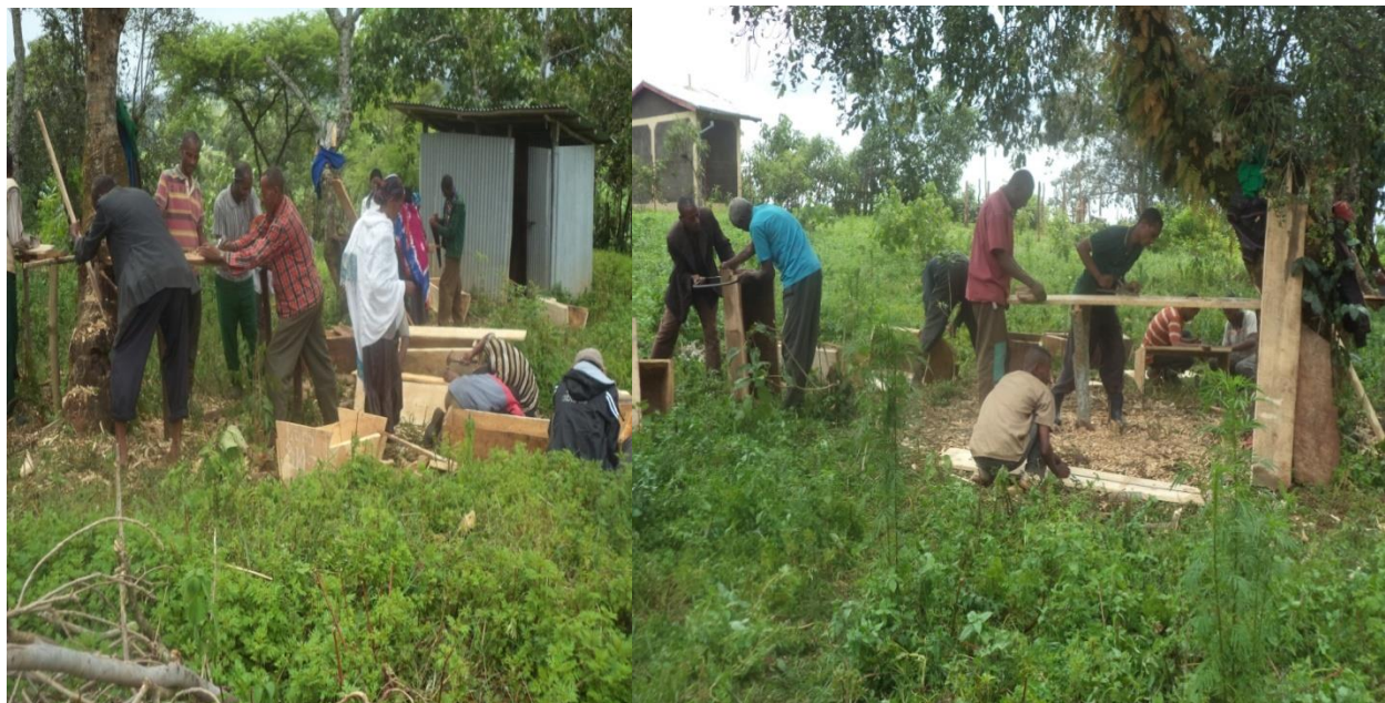
Plate 4.3.1(a) Transitional Hives Support by Self Construction
