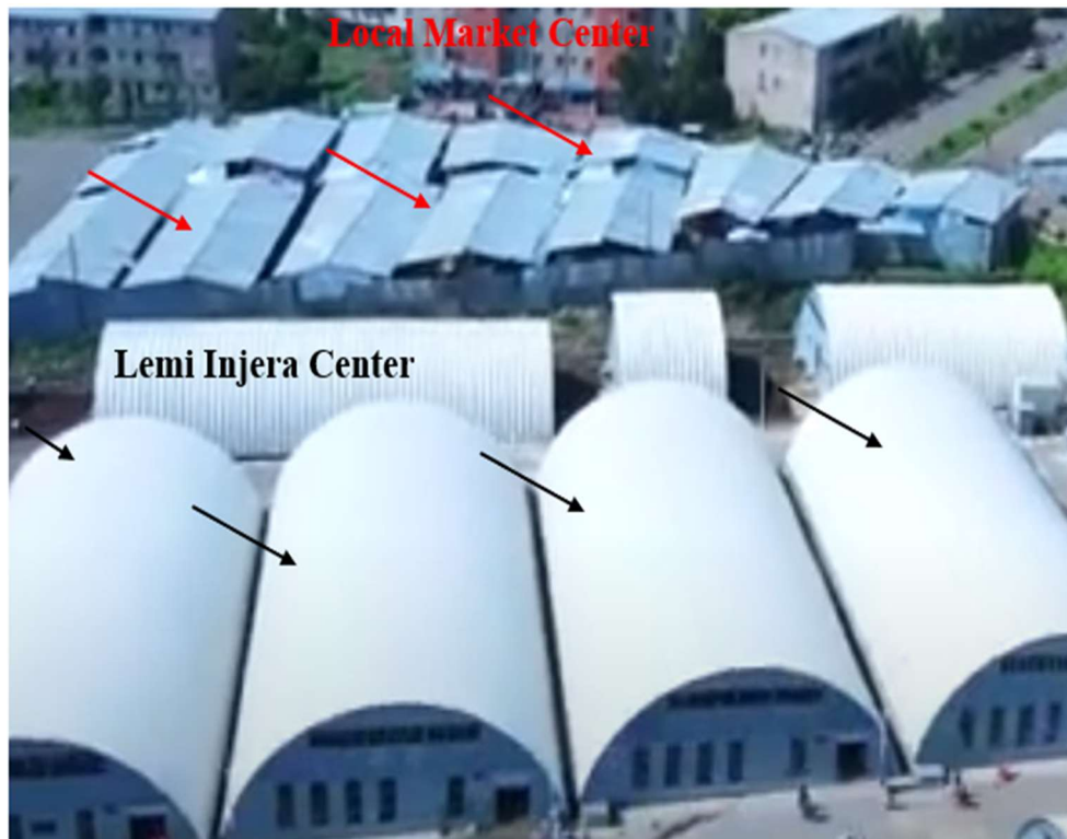
Figure 7: Study area: Image of Baking and Local Market, Lemi Kura, Addis Ababa.
