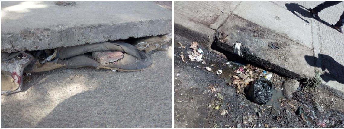
Figure 3.11: Covered manhole entry points
