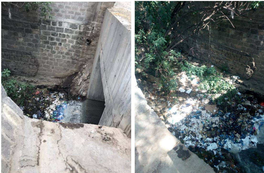
Figure 5.6: Collection of rubbish in the upstream of existing culvert
