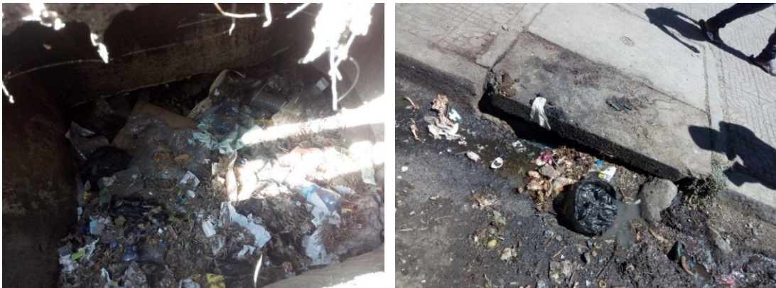
Figure 5.5: Collection of rubbish in the manhole (Source: Nefsi silk2 station)
