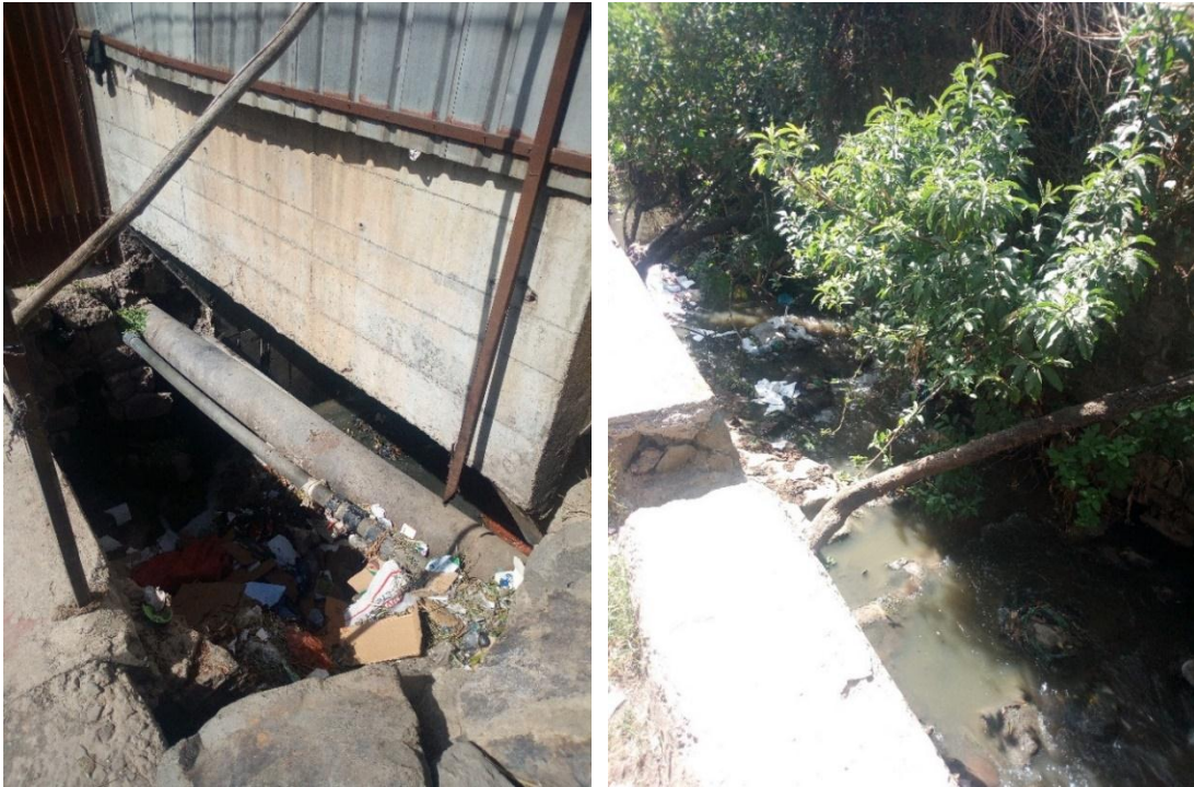
Figure 5.6: Collection of rubbish in the upstream of existing culvert
