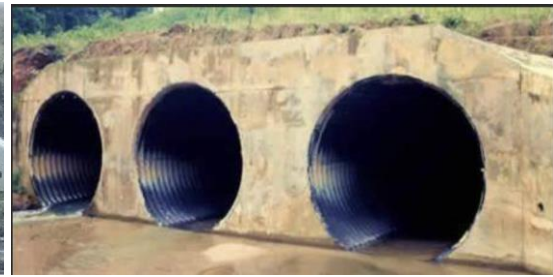
Corrugated steel pipe culvert
