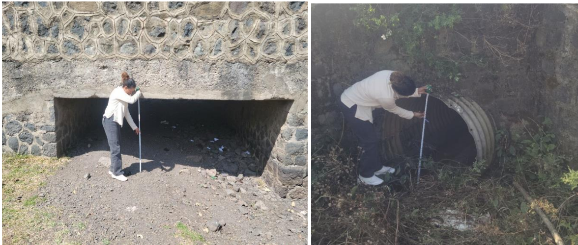
Figure 4-18: Sample drainage structure from the study area
