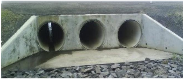
Reinforced concrete pipe culvert
