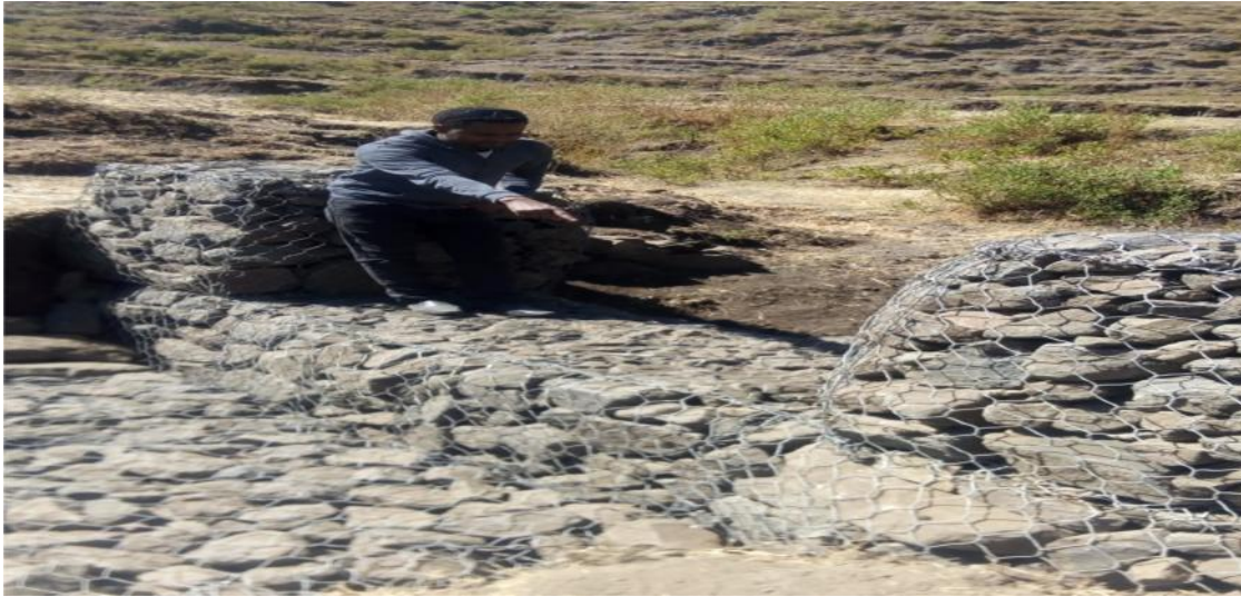
Figure 12: Gully treatment done by BOARD in Keren Awulie
