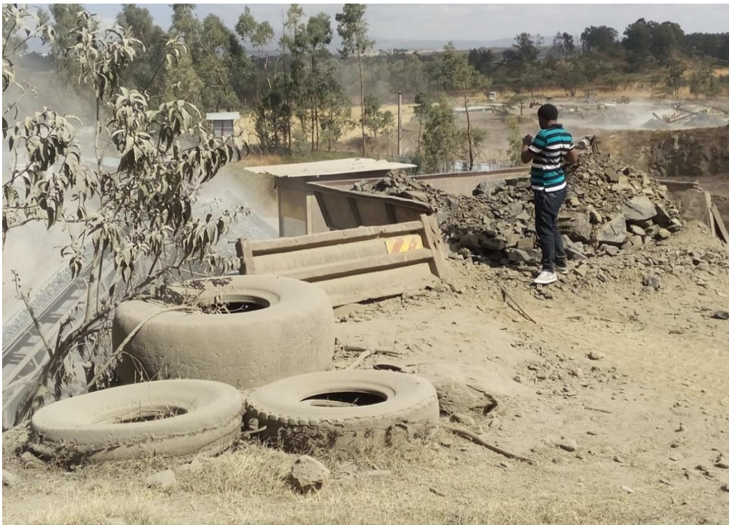
I-2: Crusher site where BCD1 (crusher dust with 20% clay) is produced due to less scalping
