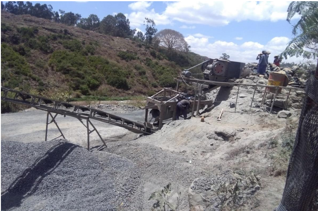
I-1: Crusher site where BCD2 (pure basalt powder) is produced due to proper scalping of parent rock
