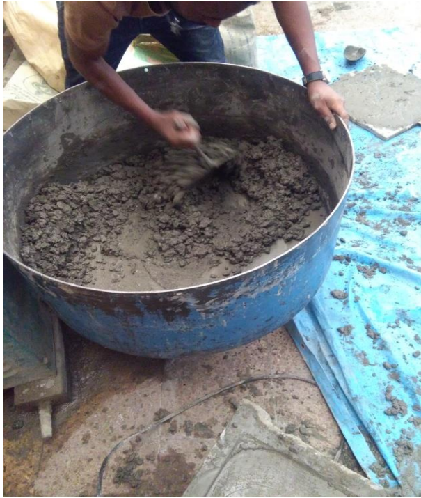
I-11: Concrete mixing
