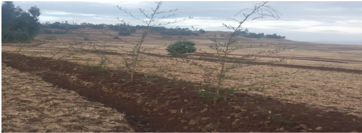
c). Construction of soil bund integrated with biological conservation
