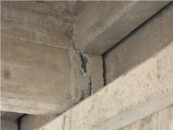
Figure 3-11 Shear crack on C100-1-045 River Bridge
