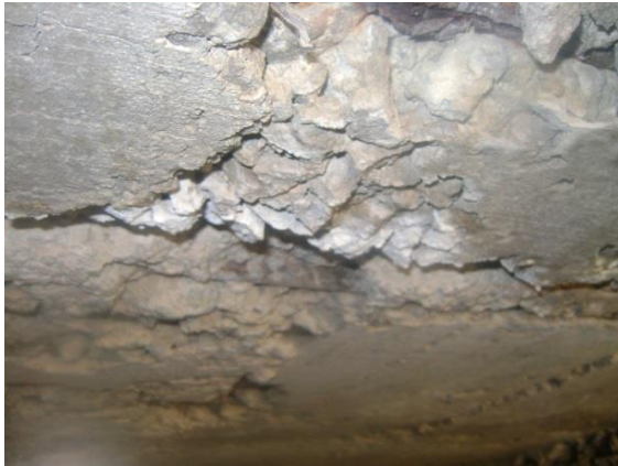
Figure 3-4 Corrosion and spaling damages on A1-1-006 River Bridge
