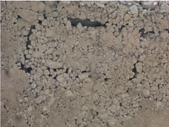
Figure 3-10 honey comb on C100-1-042 River Bridge
