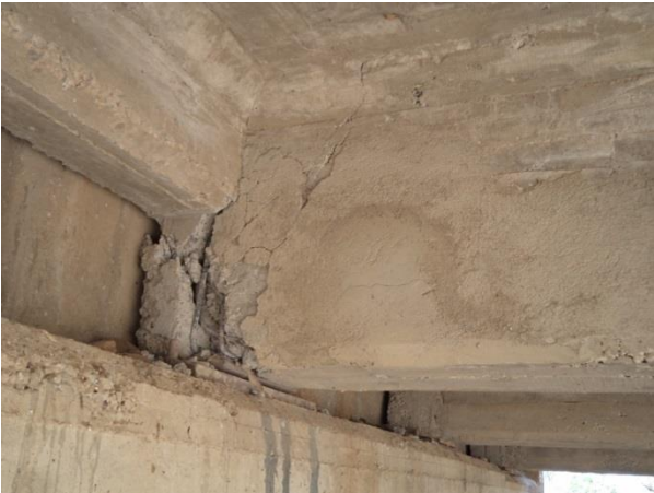
Figure 3-7 Shear crack on C100-1-003 River Bridge
