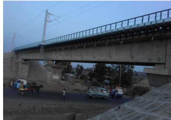
Figure 4-3: Ballasted Track Bridge in Adama city, Ethiopia
