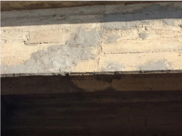
Figure 3-5 Peel off, Corrosion and Hony Comb on A1-1-007 river Bridge
