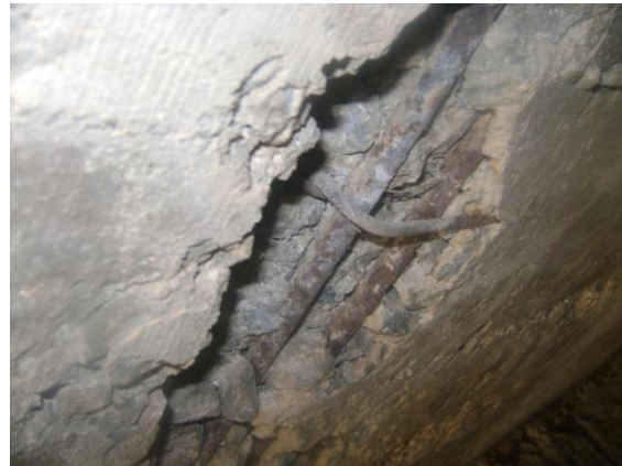
Figure 3-4 Corrosion and spaling damages on A1-1-006 River Bridge
