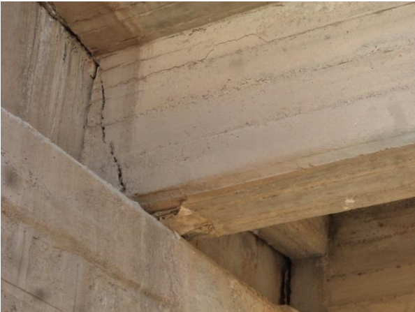
Figure 3-7 Shear crack on C100-1-003 River Bridge
