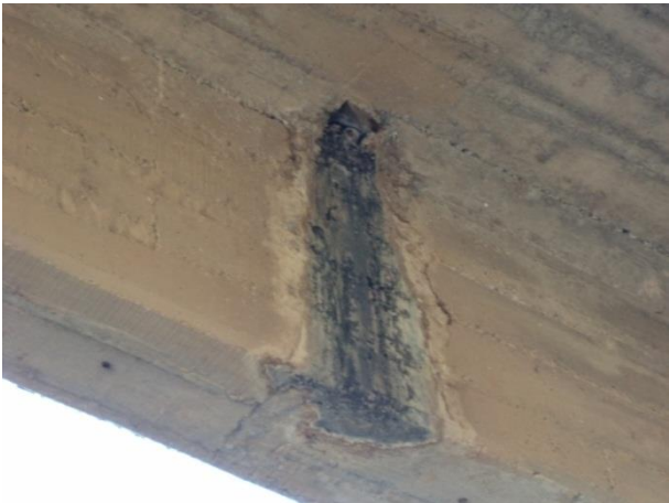
Figure 3-6 Water leakage and crack on A10-1-018 River Bridge
