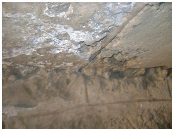
Figure 3-4 Corrosion and spaling damages on A1-1-006 River Bridge
