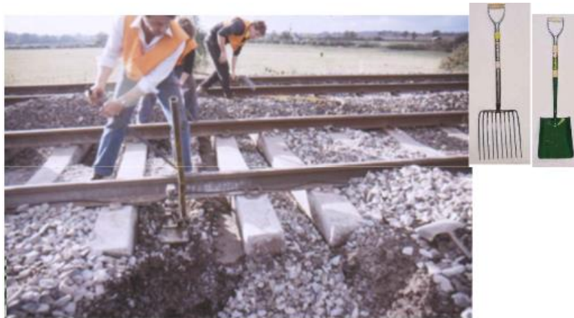
Figure 4-5 Manual renewal of ballast
