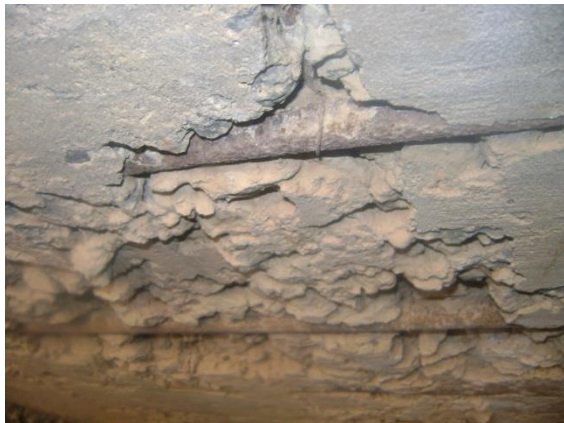
Figure 3-4 Corrosion and spaling damages on A1-1-006 River Bridge
