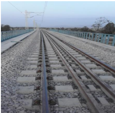
Figure 4-3: Ballasted Track Bridge in Adama city, Ethiopia
