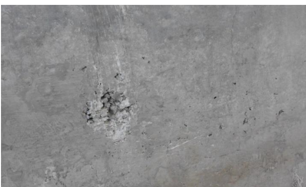
Figure 3-13: Photographs shows Crack, spalling and honey comb on Ayat terminal station bridge
