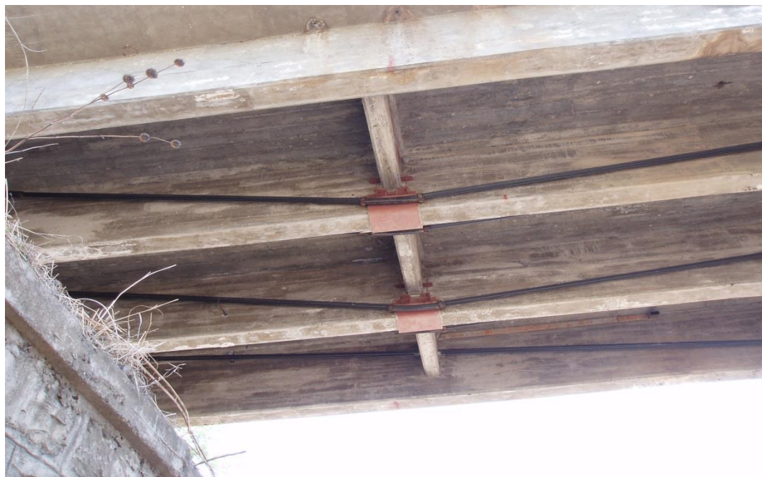
Figure 5-2 The Gibe River Bridge strengthen cable configurations
