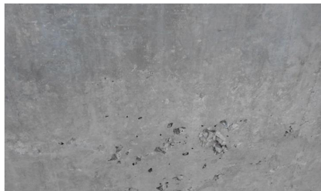
Figure 3-13: Photographs shows Crack, spalling and honey comb on Ayat terminal station bridge
