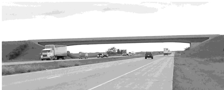
Figure 2-3: Anchored end span bridge located in north-central Illinois
