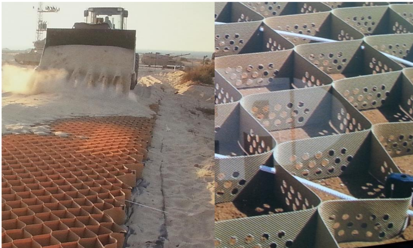
Figure 6.1 Geocell cellular confinement
