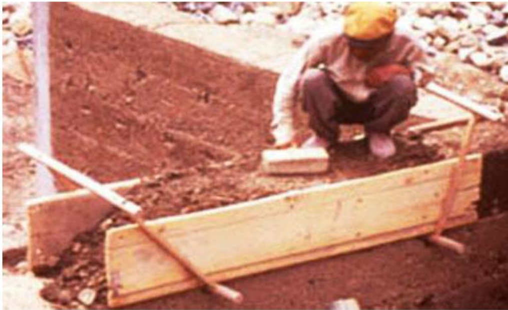
Figure.2.5. manual rammed earth technique, india[18]
