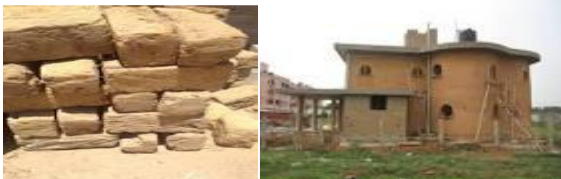
Fig.2.9. Cob and cob house in India
