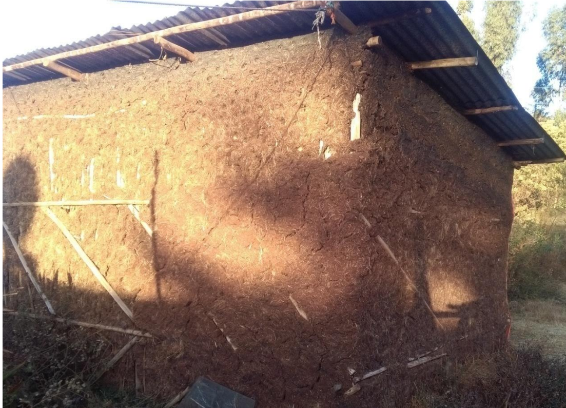
Fig.2.2. Traditional mud house building in Ethiopia
