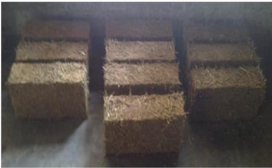
Fig.2.7.compacted, casted Mud block plastering over Straw-bundle [4]
