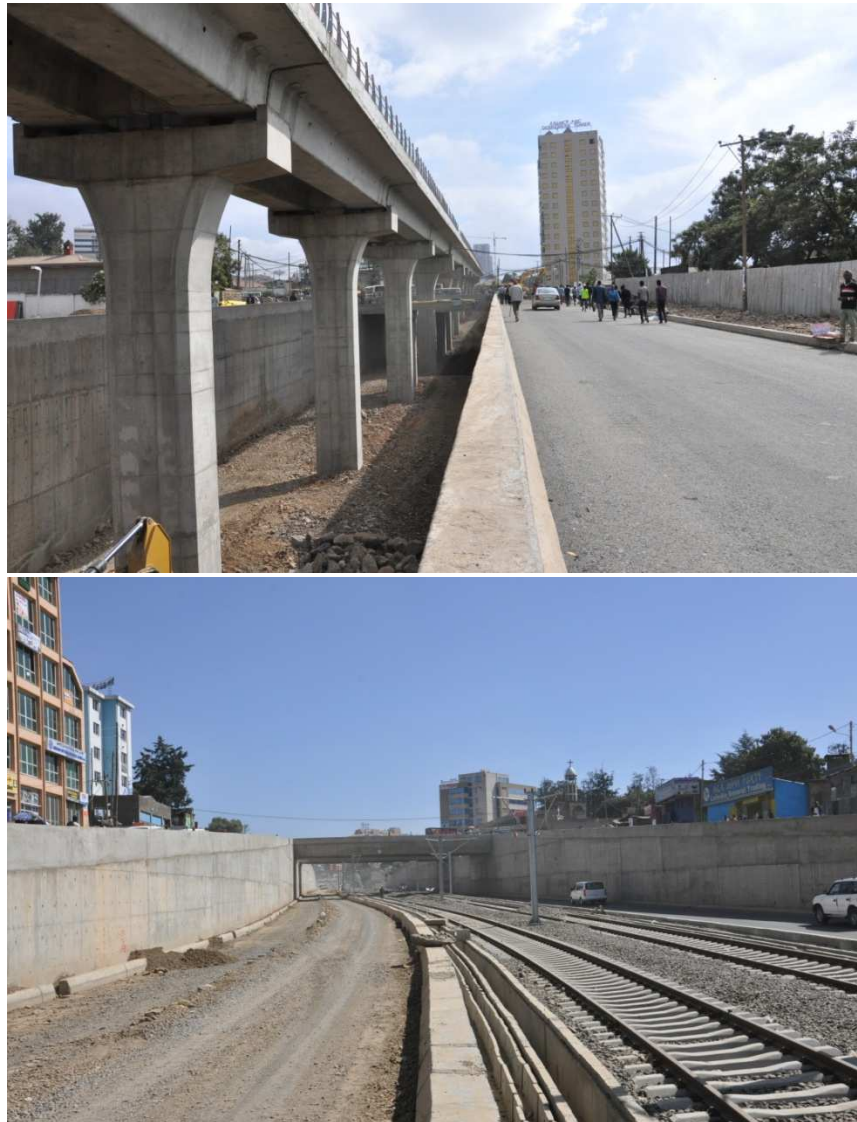
Figure 4.3: Elevated and Underpass Section of the Railway.
