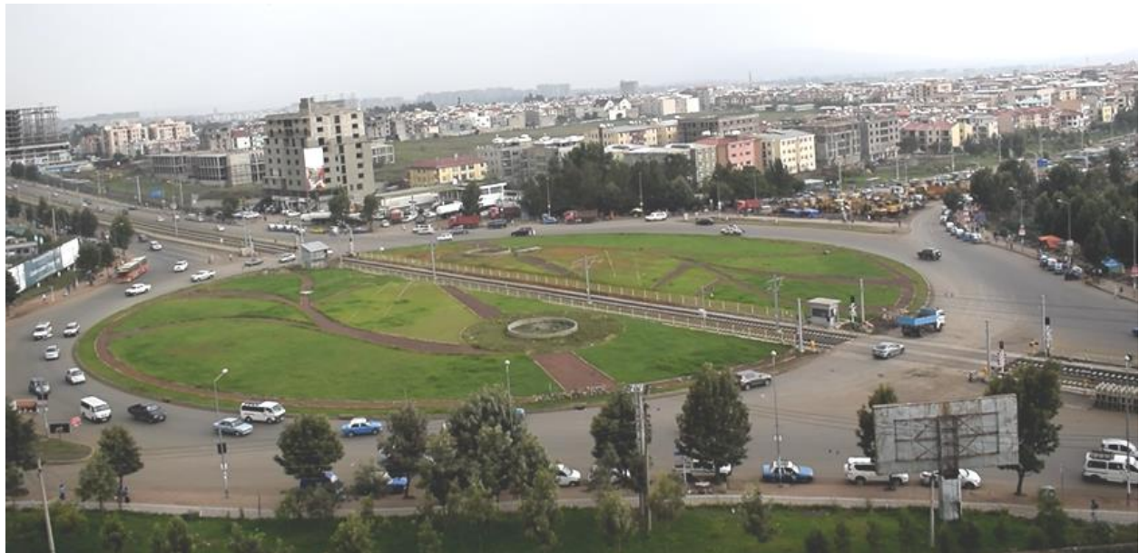
Figure 59 Off - peak traffic of CMC roundabout
