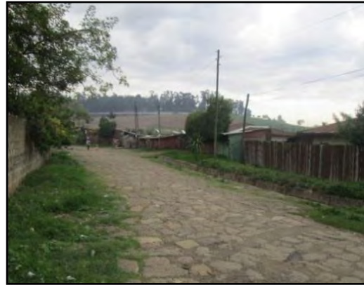
Figure 4.14: Common Road in sample area
