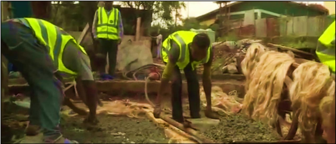
Figure 7: Manufacturing process of precast elements
