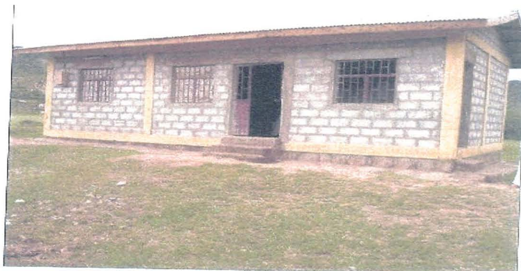
Figure 4: Women Resource Center in Yabello District Constructed by AFD
