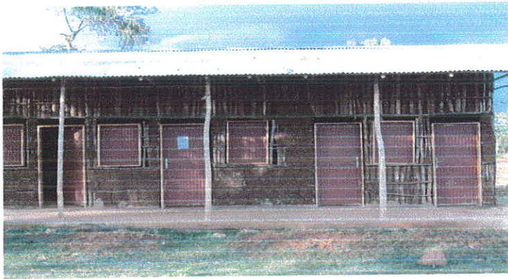
Figure 4.4: Health post under construction
