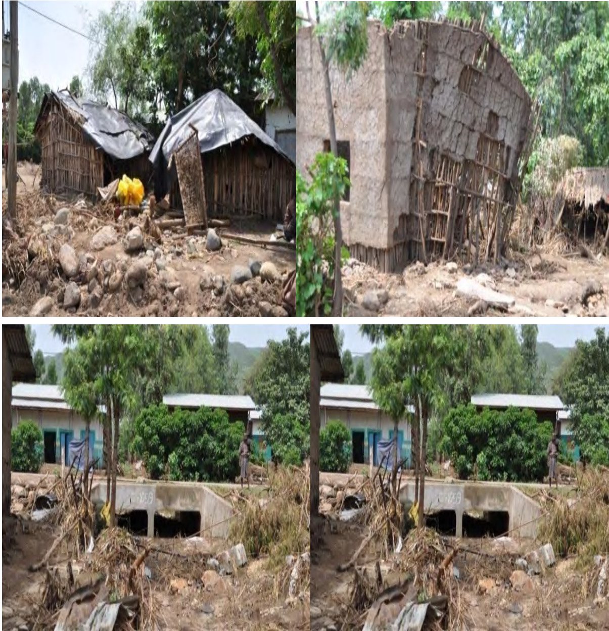
Figure 1-1: Pictures showing small part of the night of 10 August 2013 damages.
