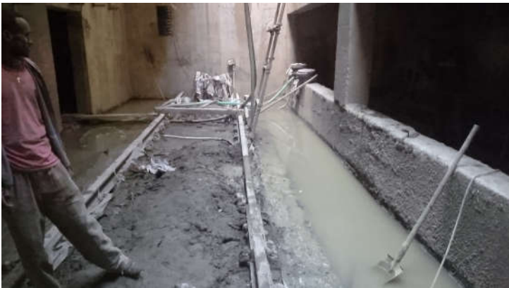
Figure 7 Tunnel start water pumping
