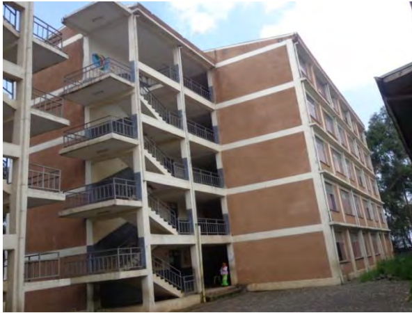
Photo 4.4 G+4 School Building
