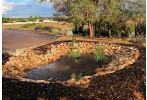
Figure 3.6 Bio-retention System
