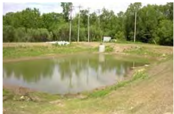
Figure 3.8 Sedimentation Basin
