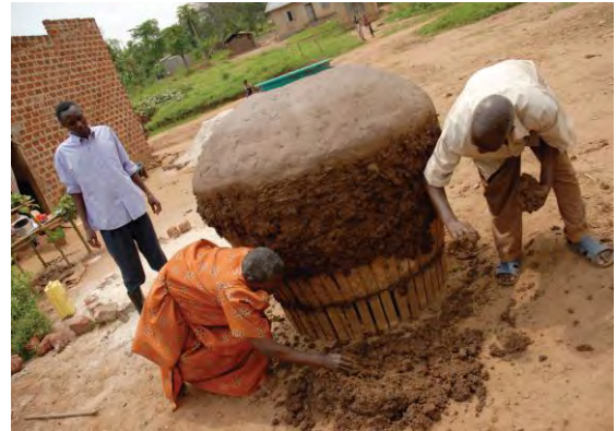
Figure 3.16 Anna Maria Nanvubya and Husband Zevilo Constructing a Rainwater Harvesting Jar at their Home in Kitayita Village.
