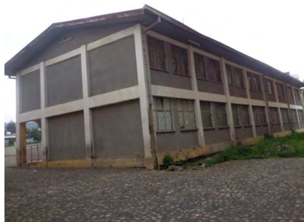
Photo 4.5 G+1 Administration Office
