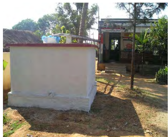
Figure 3.15 A Clean Storage Tank on a Painted White on the Outside Platform
