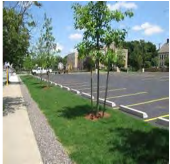
Figure 3.11 Infiltration Trenches
