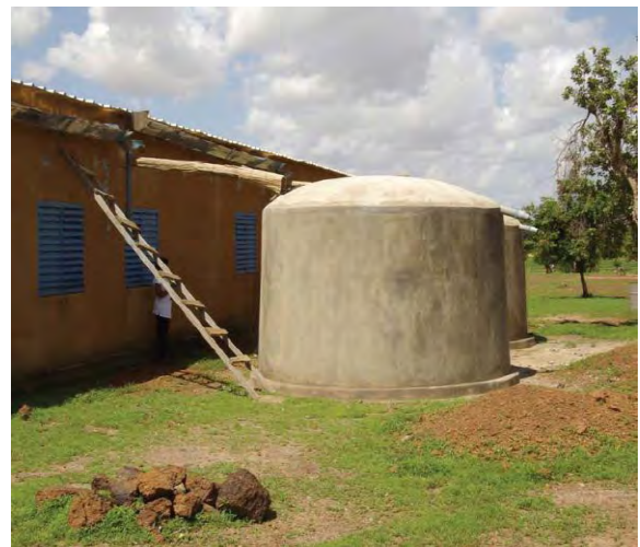
Figure 3.17 A Rainwater Harvesting Tank at a School Guirhora kello.
