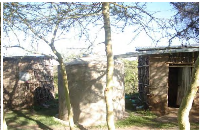
Figure 3.2 Ferro Cement Reservoir in Chele Primary School
