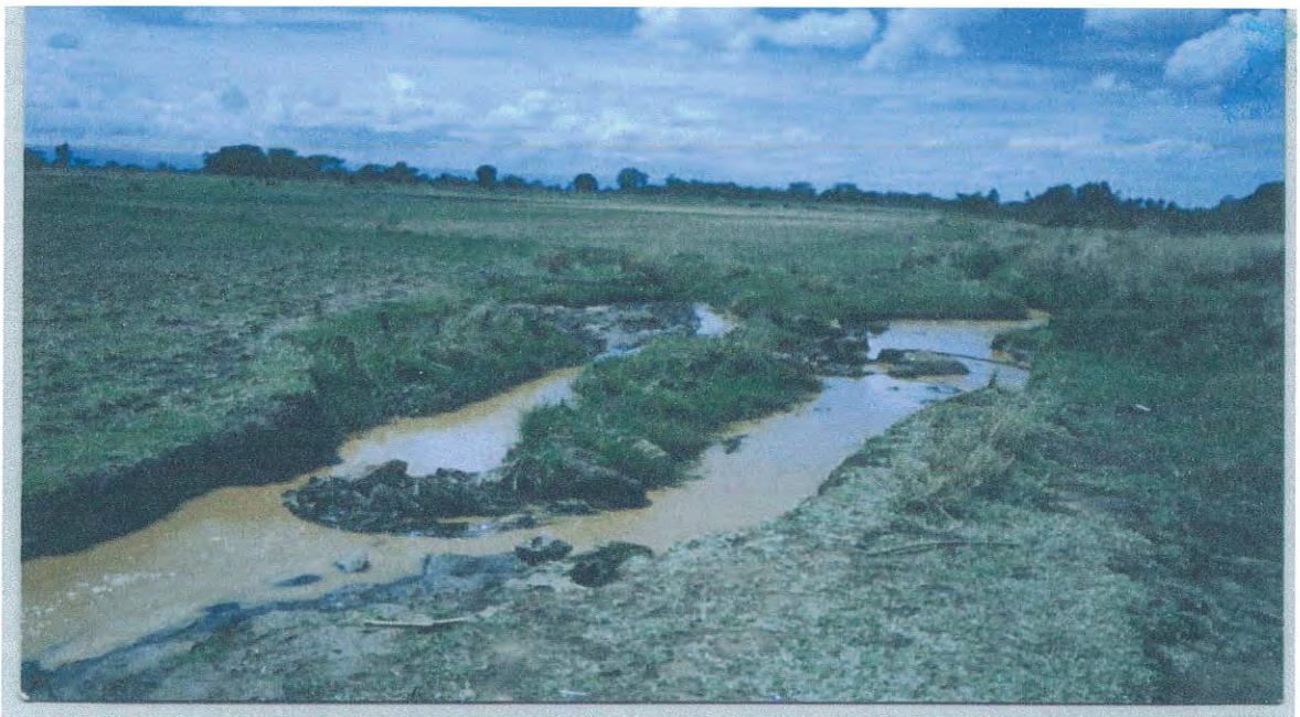
Photo 4.2: division Structure of Channel to Wandimtu Sefer
