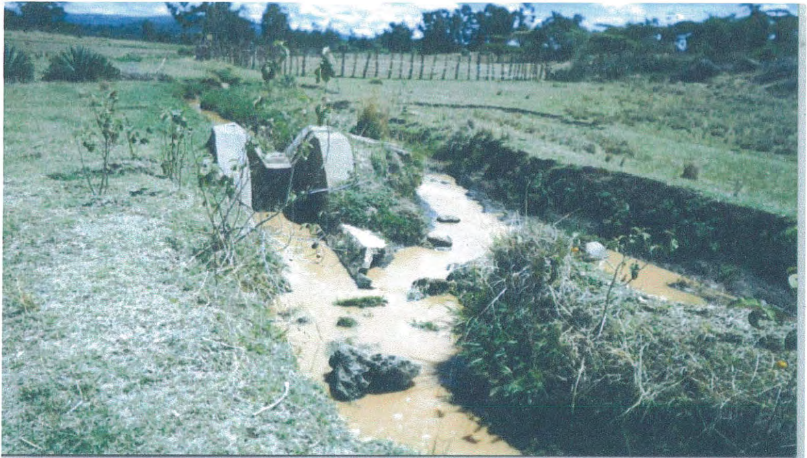
Photo 4.1: Dropping Structure of the Main Canal
