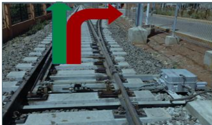
Figure 3-3: Switch and Point machine [42]
