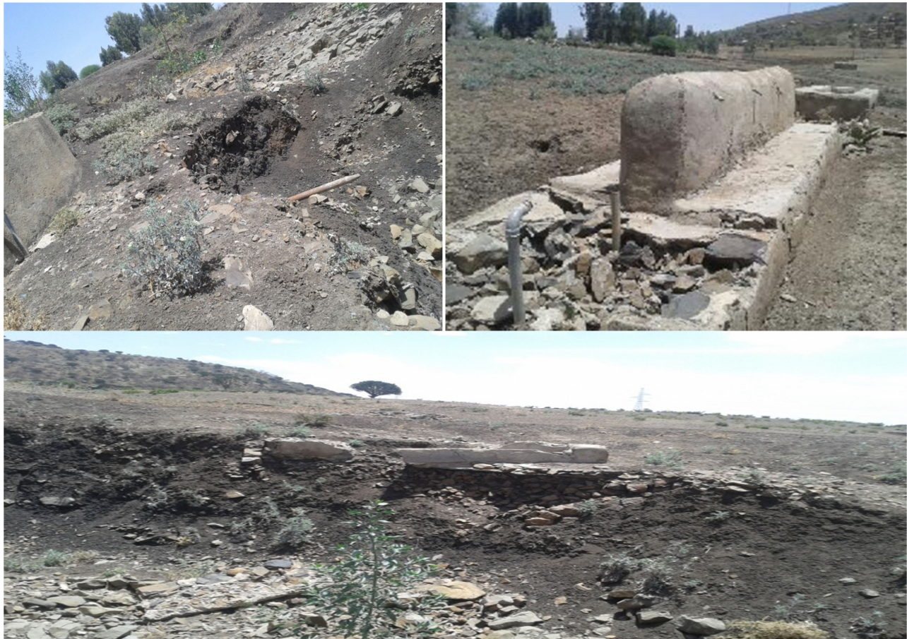
Figure 4.32 Failed spring because of miss high flood level consideration
