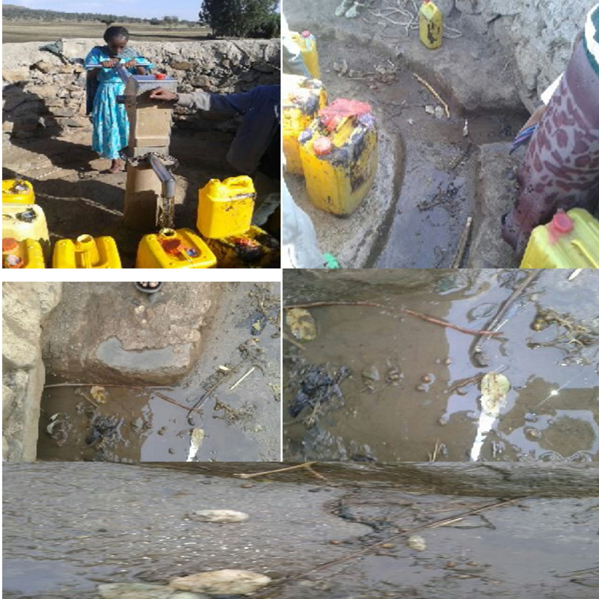
Figure 4.28 Poor drainage quality of SHW
