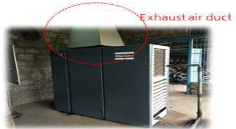
Figure 4-7: Installation of exhausted air duct at air compressor
