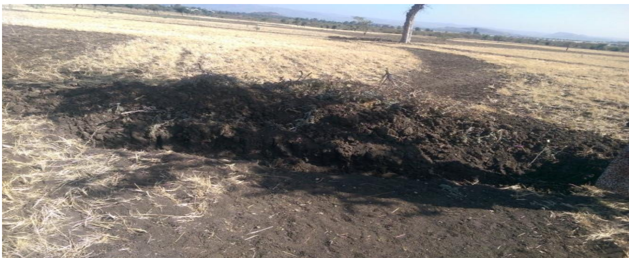
Figure 23 : Soil bund constructed by farmers with the help of development agents
