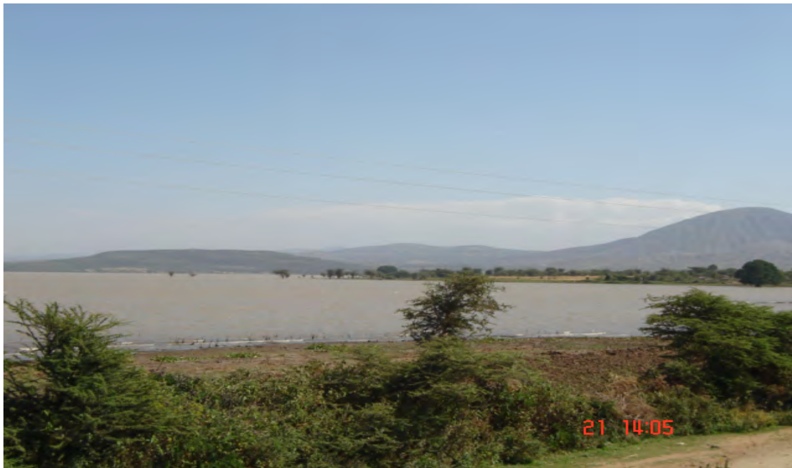
Photo 4.2 Partial View of Koka Dam
