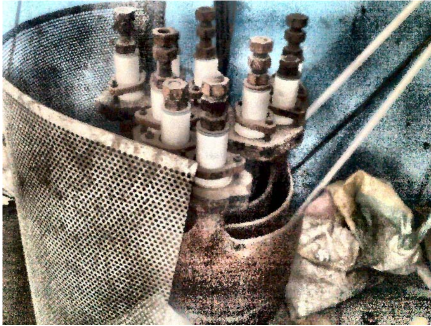
Fig.29 Heating element of the old boiler
