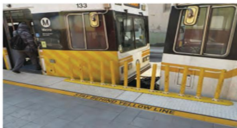
Figure 2-6: Between-car barriers flexible delineators
