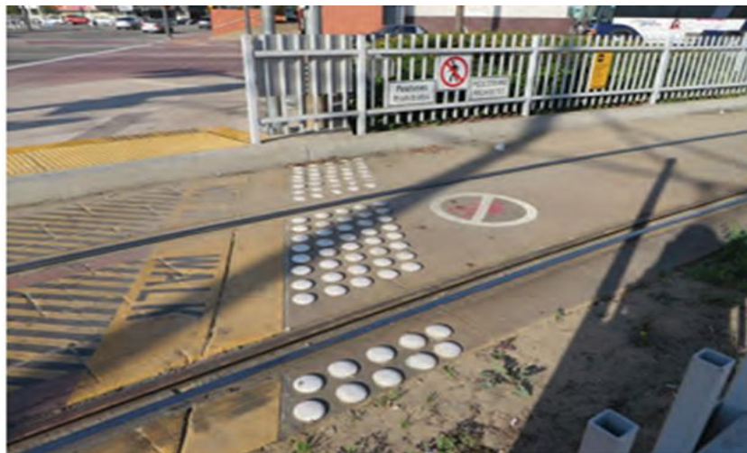
Figure 2-9: Treatments used at the station entrance
