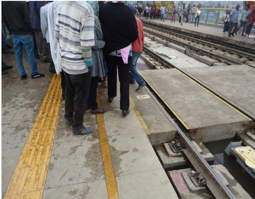
Figure 4-6: Passengers stand very close to the edge of platform (Stadium)
