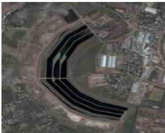
Figure 3.1: Satellite image of Kaliti wastewater treatment plant.
