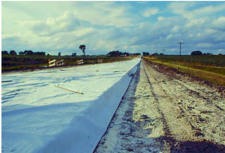
Figure 8- Insulating blankets in place on freshly-placed concrete
