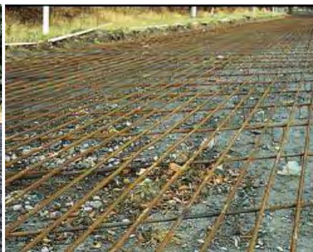
Figure 4-Improper prepared subgrade
