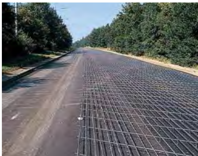
Figure 3- Carefully prepared subgrade
