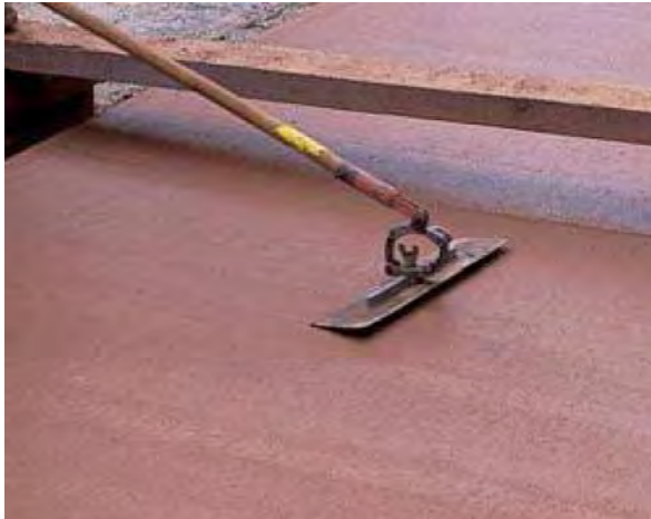
Figure 7-Concrete Finishing with Hand tool
