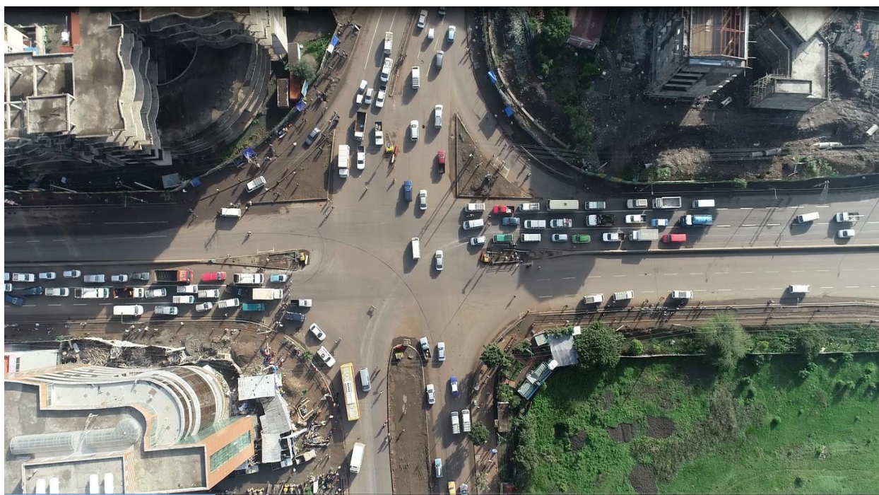
Figure 3.2: Jemo Michael Signalized Intersection
