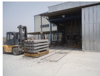
f) Sleeper taken to steam curing and storage
