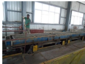
d) Concrete casting
