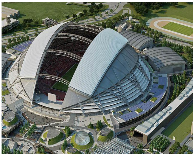
A. Singapore National Stadium
